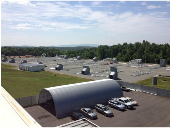
Figure 3: VRC New Indoor Area Construction Underway
