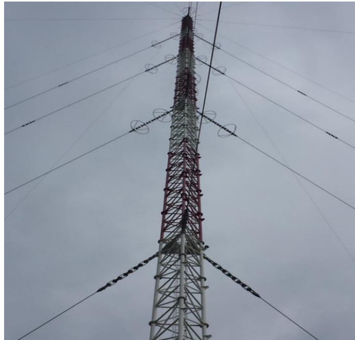
Figure 2. Single umbrella antenna of Changhe II.
